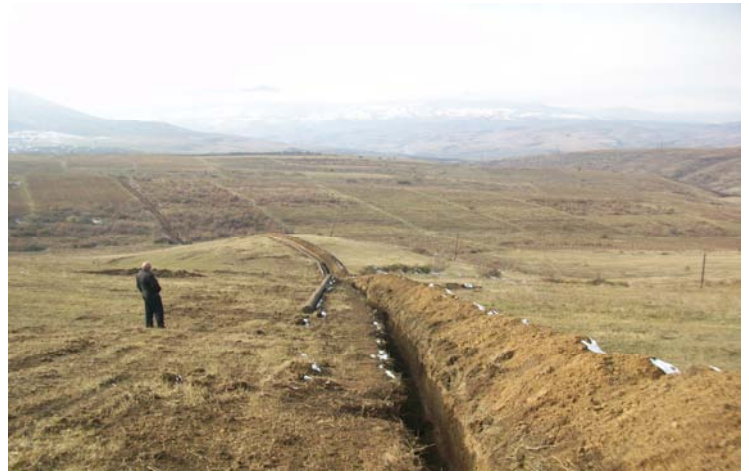
The rolling hills of the Aygehovit-Vazashen Irrigation Canal
